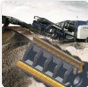
6 - Crushing and mixing
