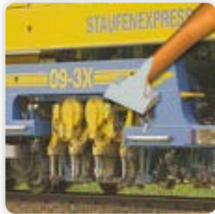
14 - Rail track construction
