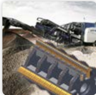
6 - Crushing and mixing
