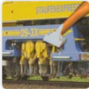
14 - Rail track construction
